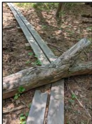
"Before" photos of broken bridge boards and fallen tree damage to a boardwalk.
