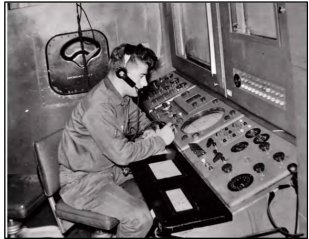
The Control Room, manned all day, every day, coordinated the signals from the varied equipment and also had the "fire" buttons. (Burlington installation) 2
