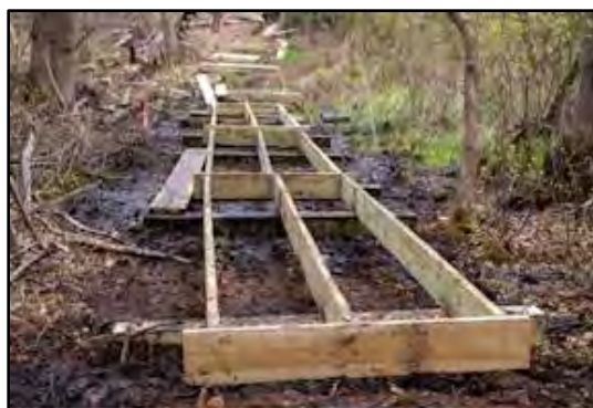
Framing is set in place over the boggy path.
