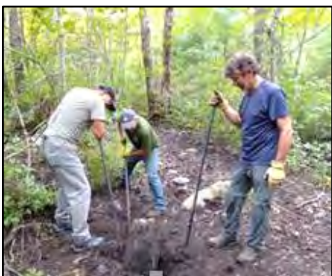
Forester Mike Labossiere, center, and SEM members Paul Audet and Larry Petrone work on the new loop trail.
