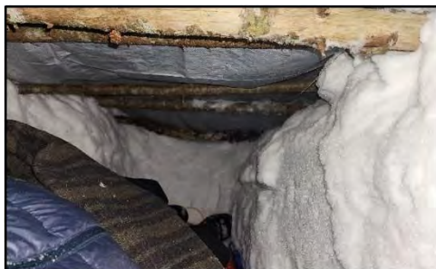
21. Ready for occupancy. Photo by Paul Brookes
