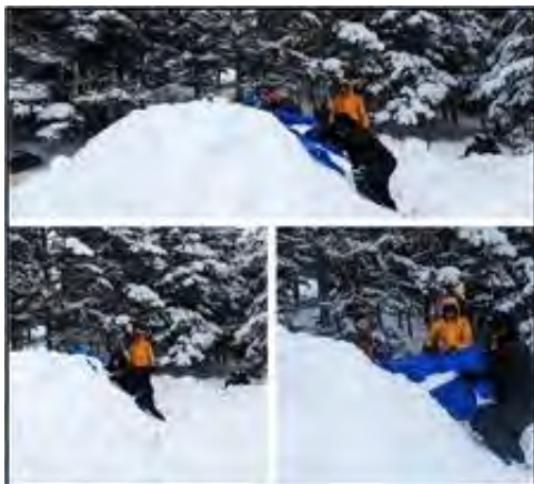
5. To build a quinzee- first pile up the snow and let it set for 45-60 minutes. The longer the better. We used shovels, helped by piling snow on tarps and dumping it on. Snowshoes can be used for digging if you don't have shovels
