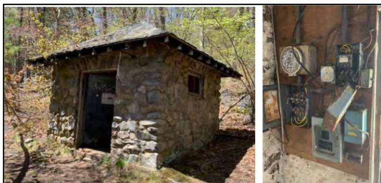
Pumphouse built in 1913 with disused electrical panel.
