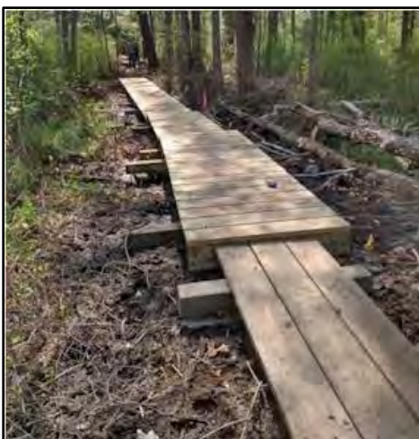
Crossboards are securely attached to the frames. Photo by Stephanie Merrill
