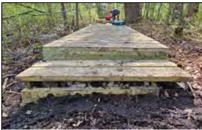
Crossboards are securely attached to the frames. Photo by Stephanie Merrill
