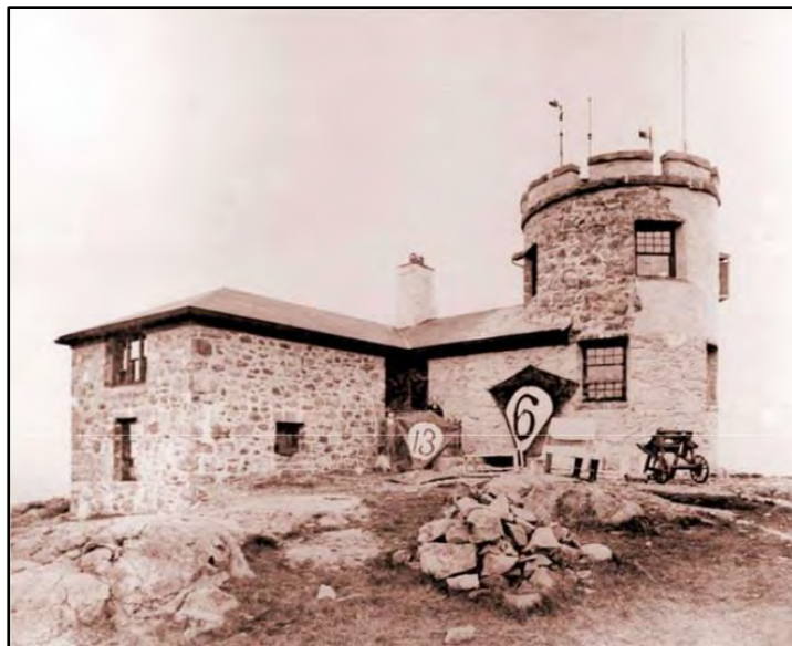
Original Observatory, in 1887, with two of the kites that were used to raise instruments into the sky. 2
