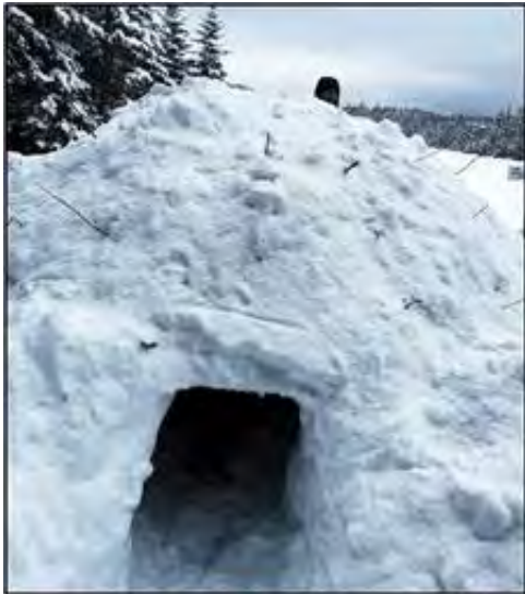
11. Foot long Twigs are put into the sides so when digging out you know when you are getting too close to the outside. Photo by Ann Hargleroad
