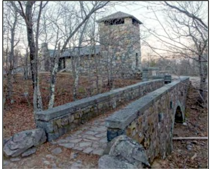
The Eliot Tower and connecting Bridge in the Blue Hills.
