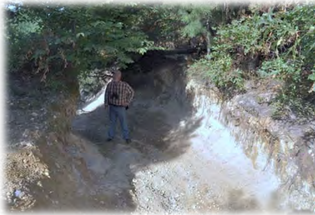
ORV and erosion damage at Freetown State Forest Photo courtesy of Everett Castro
