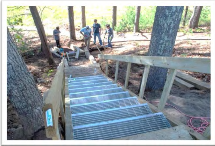
New stairs and railing provide safer access to 1623 Trail.
