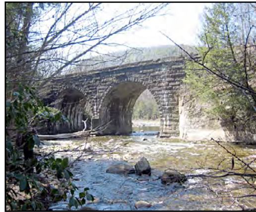
The double arch dry stone bridge. Courtesy of Len Ulbricht
