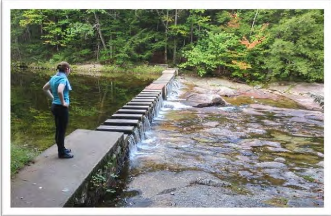
Elizabeth Robinson on the Dam over Cold River (Dexter Robinson photo)
