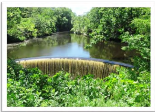
Circular weir dam at Hemlock Gorge.
