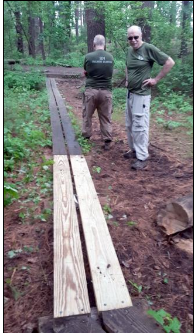
Pete Tierney inspects a section of new lumber replacing broken boards on the boardwalk.
