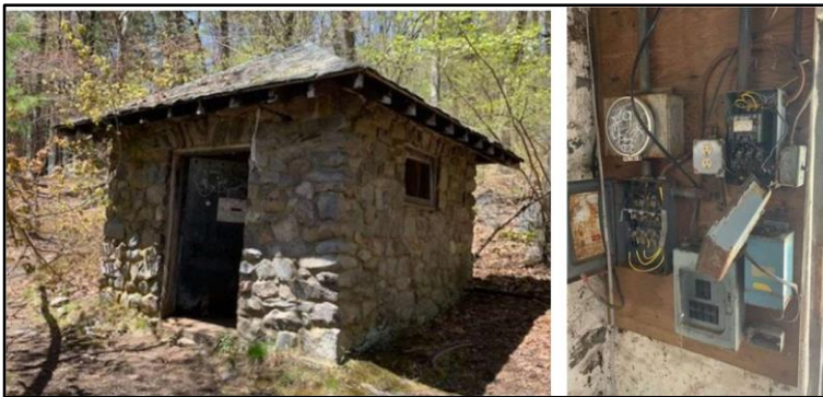
Pumphouse built in 1913 with disused electrical panel.
