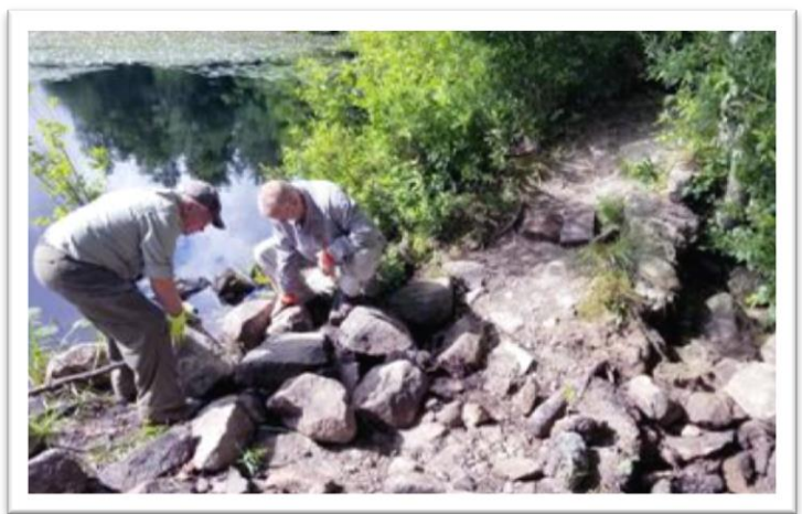
Skip Maysles, left, and Paul Brookes, right, move field stones to build the bridge abutments at both ends of the bridge span. Photo by Barry Young
