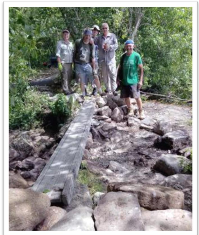
A hardy work crew constructs the fieldstone abutments at both ends of the planned new bridge. The old wooden single plank bridge in the photo will be replaced with a new wider bridge. Left to right: Skip Maysles, Bob Vogel, Pete Tierney, Paul Brookes, Charlie Farrell. Photo by Barry Young
