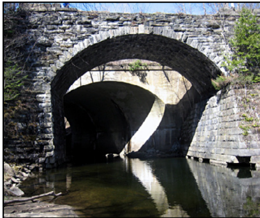
Keystone Arches Bridge with modern concrete version in background. Courtesy of Len Ulbricht
